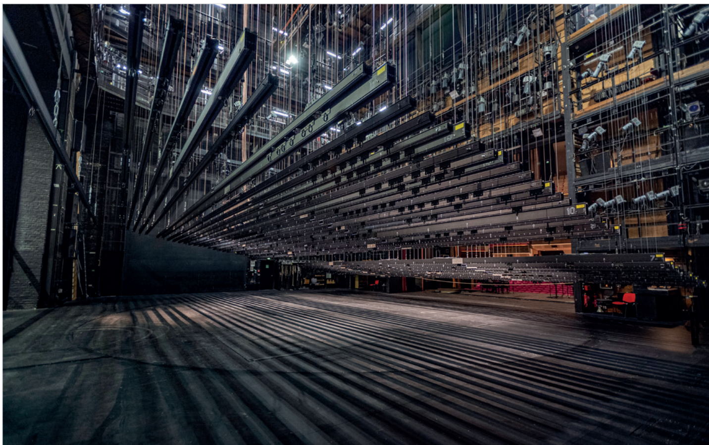
Photo: © Nasser Hashemi / Theater Chemnitz – Germany / Use of the CARGO L rail profile as a load bar for machine hoists on the main platform
