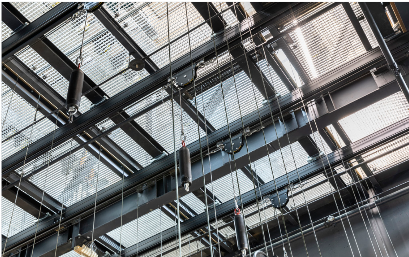
Photo: © Stephan Walzl / Oldenburg State Theater – Germany / Installation of 4 CARGO L row point hoist rails with movable outgoing roller brackets
