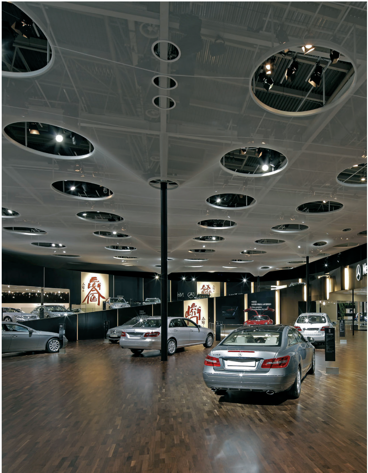
Auto China exhibition stand Mercedes-Benz – Beijing, China / Production and installation of the exhibition stand ceiling made of SPRINKLERNETZ BW exhibition textile; with oval cut-outs for the sprinker systems.
