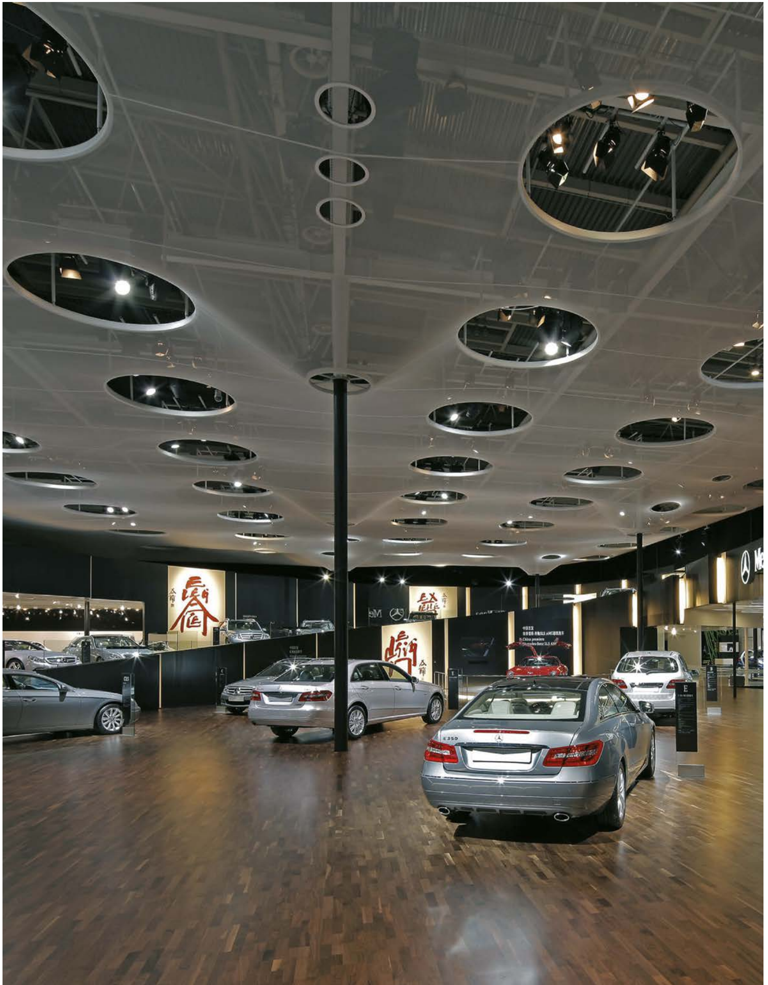
Auto China exhibition stand Mercedes-Benz – Beijing, China / Production and installation of the exhibition stand ceiling made of SPRINKLERNETZ BW exhibition textile; with oval cut-outs for the sprinkler systems.
