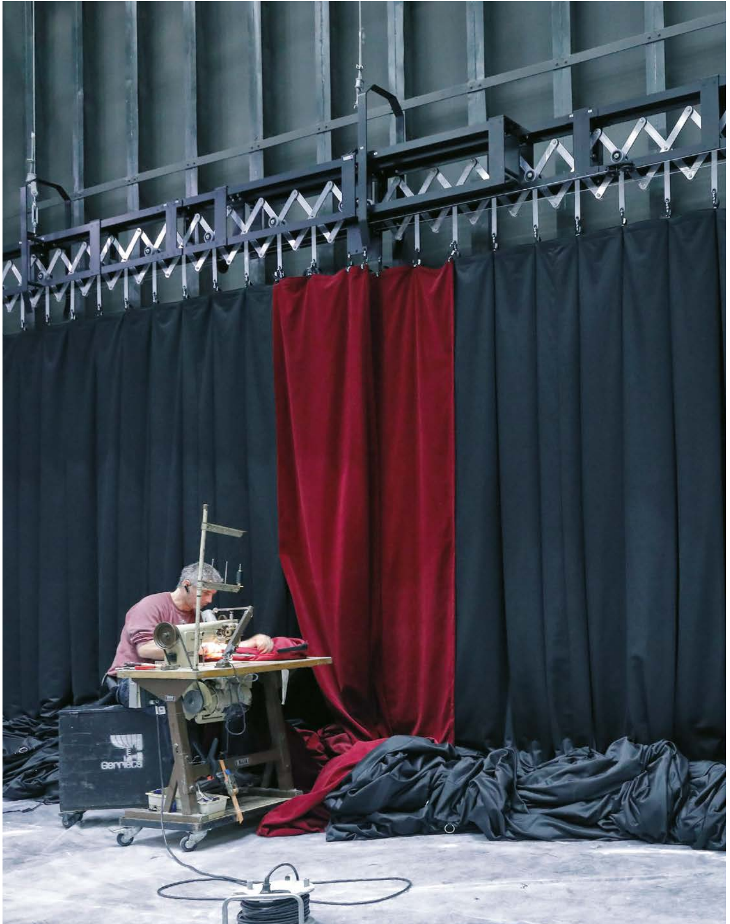
Photos: © Philipp Zinniker / Concert Theater – Bern, Switzerland / Two-part main curtain made of ALICANTE and SATIN CS on a FENCE scissor pull system
