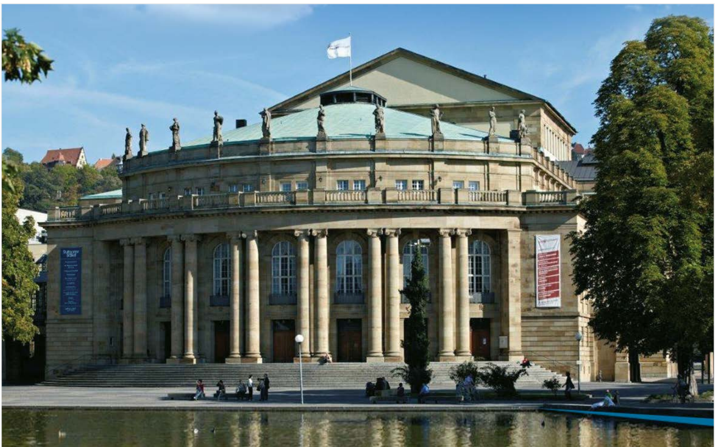
Photos: © Gerriets GmbH / State Opera – Stuttgart, Germany / FENCE scissor lift and STRATUS Roman blind systems incl. curtains made of SATIN CS
